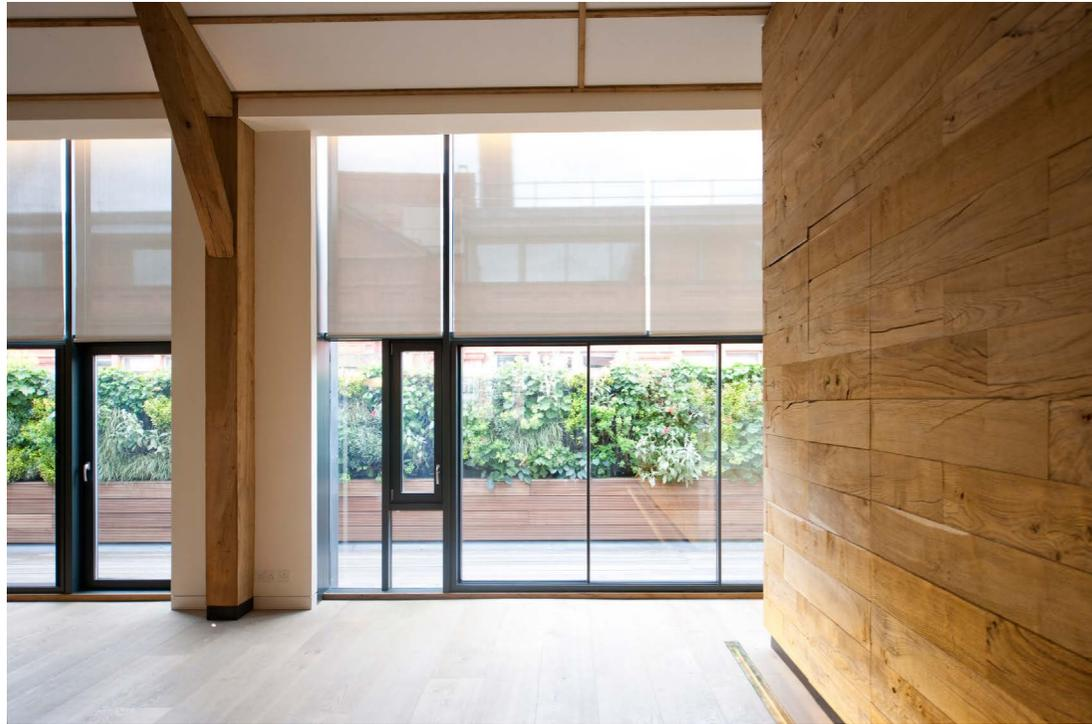
sandblasted oak beams and columns with dowelled mortise and tenon pinned joints
