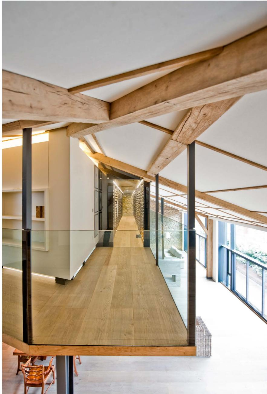
Ultra thin mezzanine floor finished in manipulated engineered oak boards- hanging off the roof
