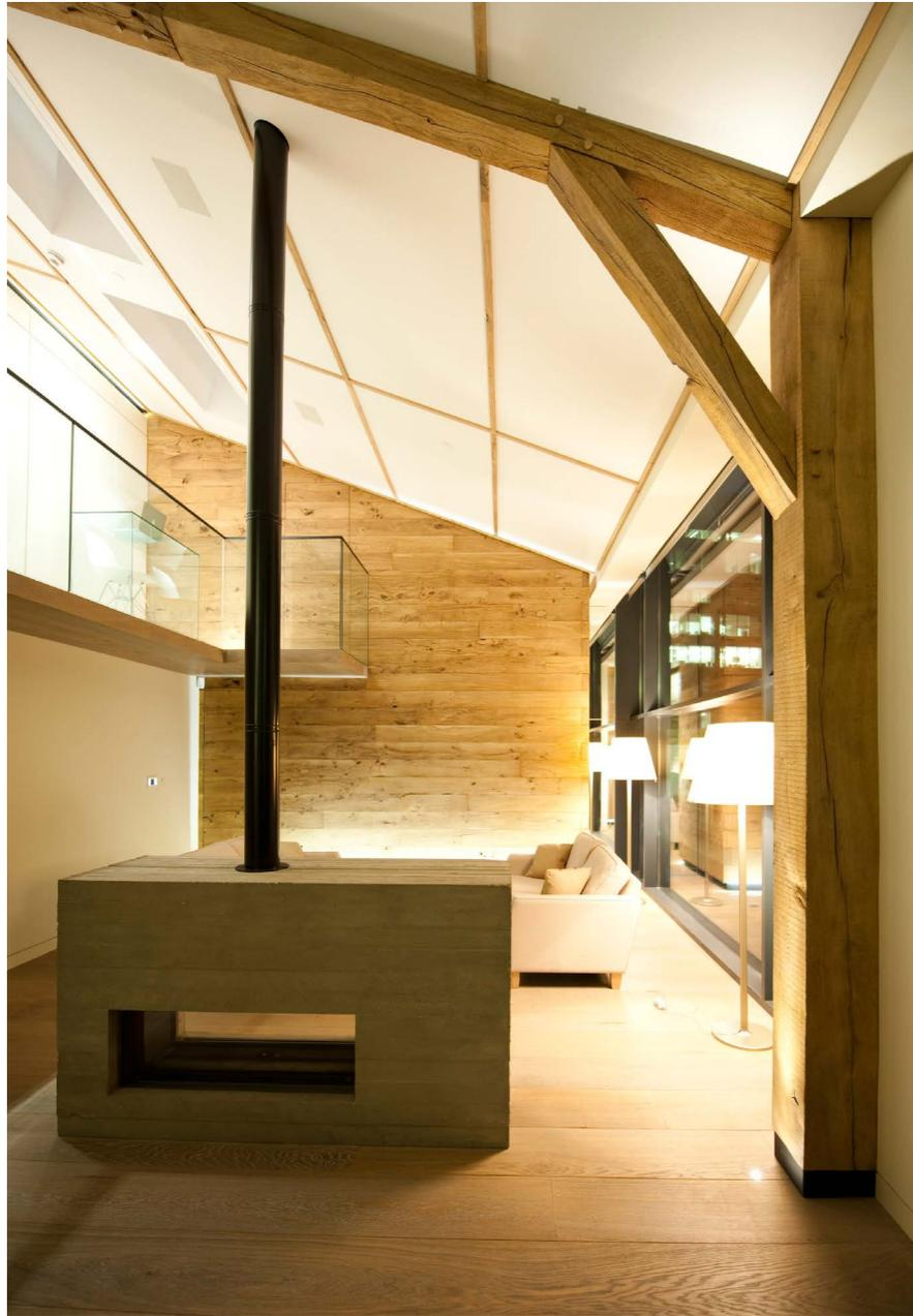
in-situ cast concrete fireplace with exposed timber plank shuttering combines both the natural concrete and natural texture of timber
