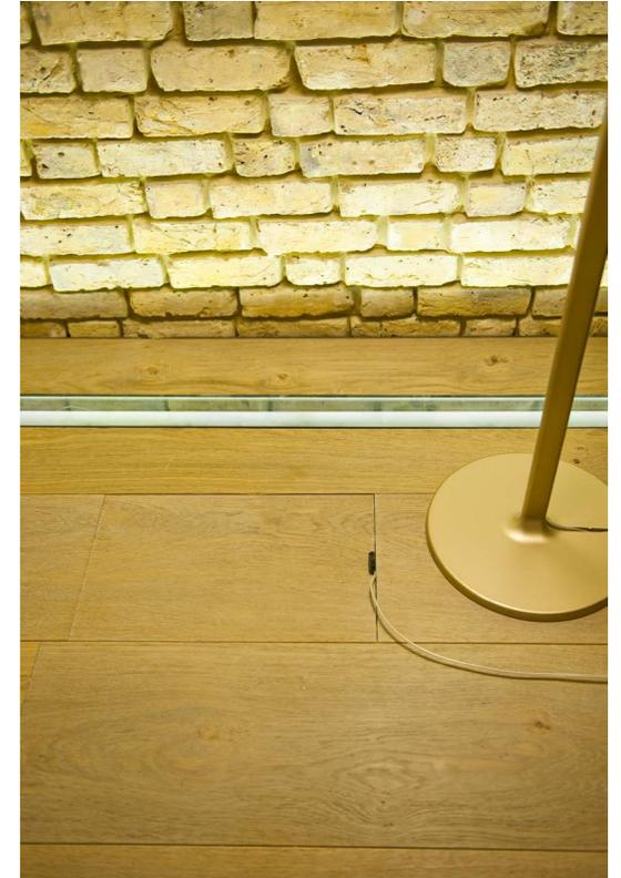
the concealed services with ethernet and telephone, power hidden in floor socket boxes to avoid visible wires at all costs
