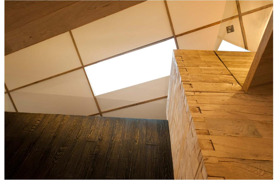
oak sections have been designed to express the depth of the sand blasted oak with an expressed 'finger' or 'comb' joining detail
