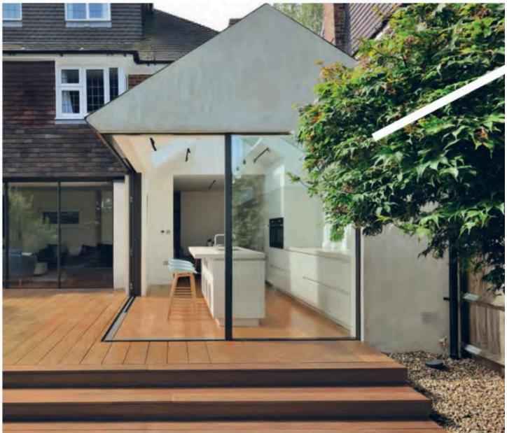
that PMA specifically developed in the studio's laboratory for this project. The facade intentionally resembles natural stone, to balance with the eco material palette of the project. Adding to the overall impact is the project's concept of bringing the 'outside in' through the design of retractable glazed sliding walls which, as they open, enable the kitchen and garden to become one.
