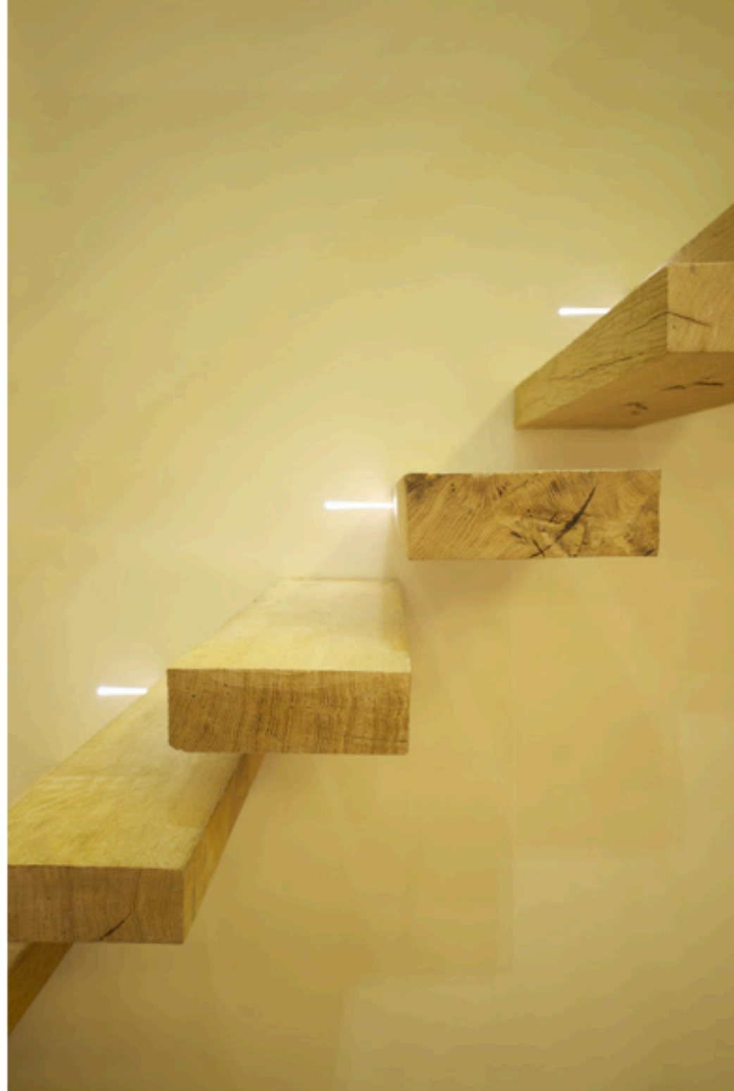
photographer: Paul McAneary Architects Ltd
