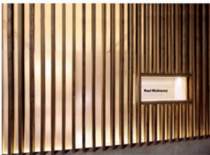
↓ The oak used for the facade was cut and shaped in the office
